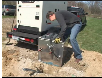
Figure 11. Place the GeoCube on Stable Ground
