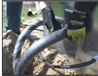
Figure 13. Insulate the Loops
