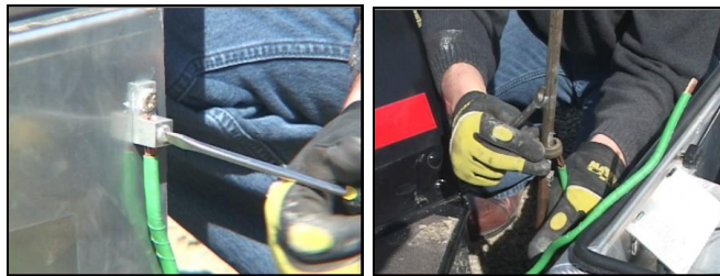
Figure 14. Grounding the GeoCube and the Generator
